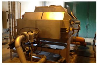
The new gravity based Alfa Laval AS-H Belt Thickener.
