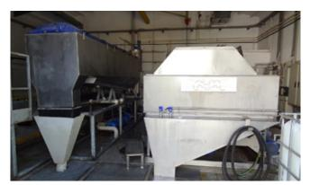
The existing rotating Alfa Laval Drum Thickener (left) and the new Alfa Laval AS-H Belt Thickener.
