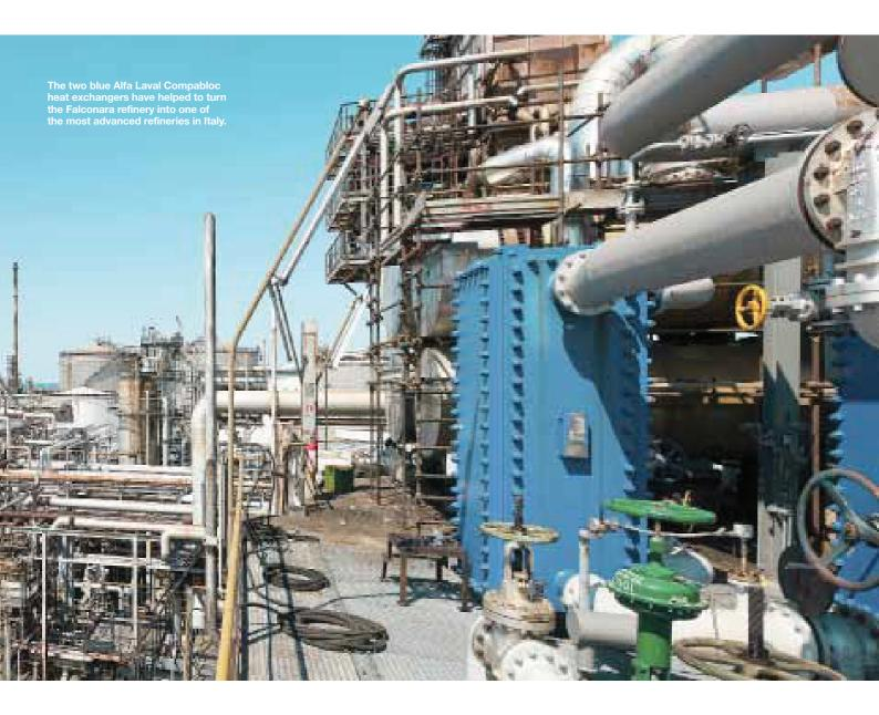
Falconara's maintenance of the second-stage overhead air coolers in the crude distillation units showed that by making changes to the system the plant could optimize the heat it produced more efficiently. Officials had the option of either replacing the damaged air coolers with the same technology or installing new but unfamiliar Alfa Laval Compabloc welded plate heat exchangers designed to recover heat otherwise wasted in that part of the refining process.
